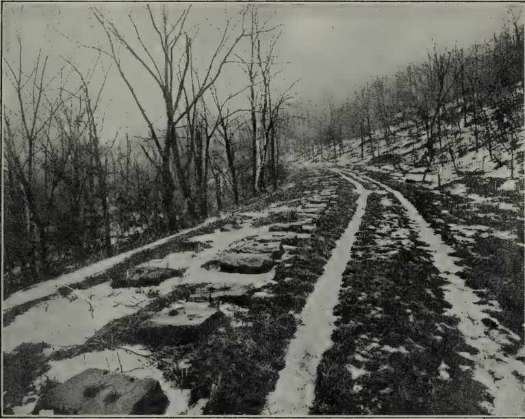
A railroad right-of-way — a bit of the roadbed of the Old Portage Railroad, near Gallitzin, Pa., showing stone sleepers which proved not to be practical.
